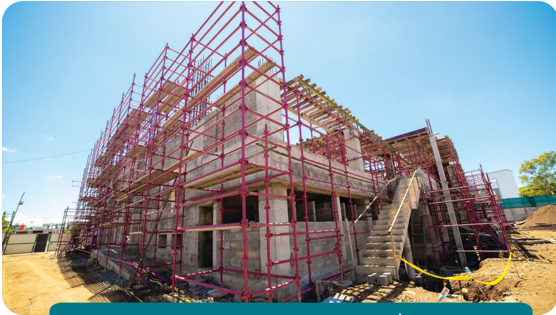
Construction of Multipurpose Sport Complex/Gymnasium at Stanley, Rose Hill
