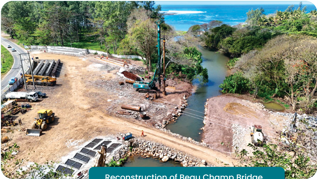
Reconstruction of Beau Champ Bridge at Bel Ombre
