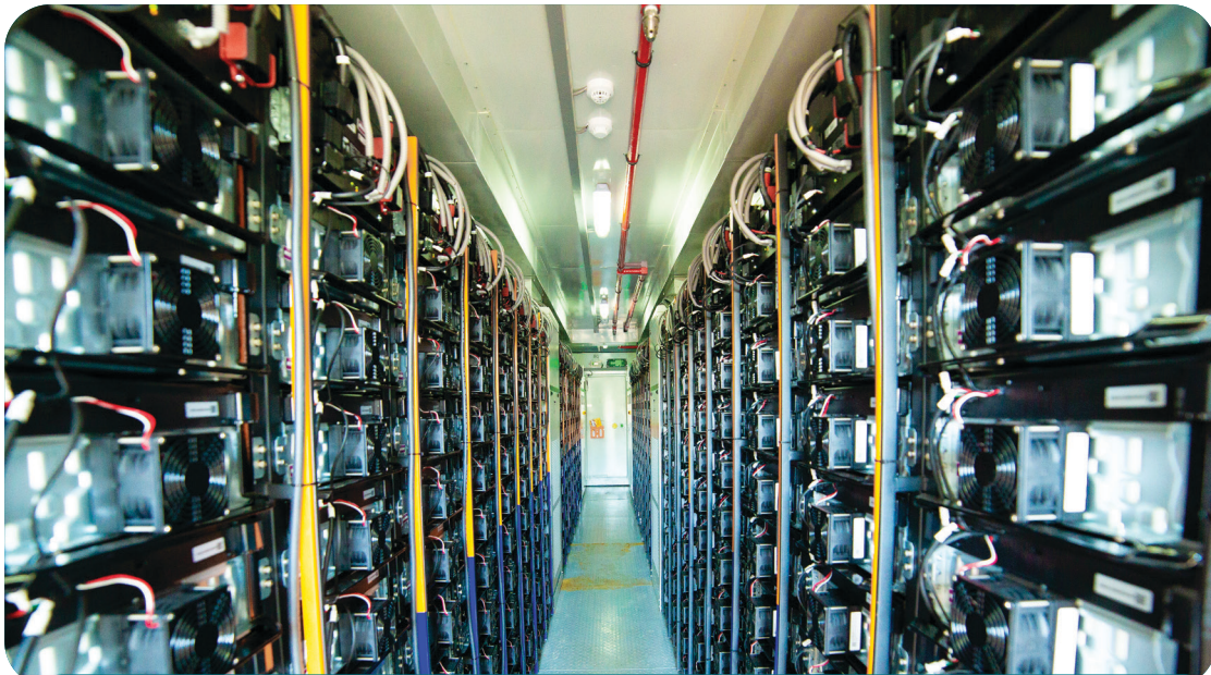
Design, Manufacture, Supply, Installation & Commissioning of a 20 MW Battery Energy Storage System (BESS)
