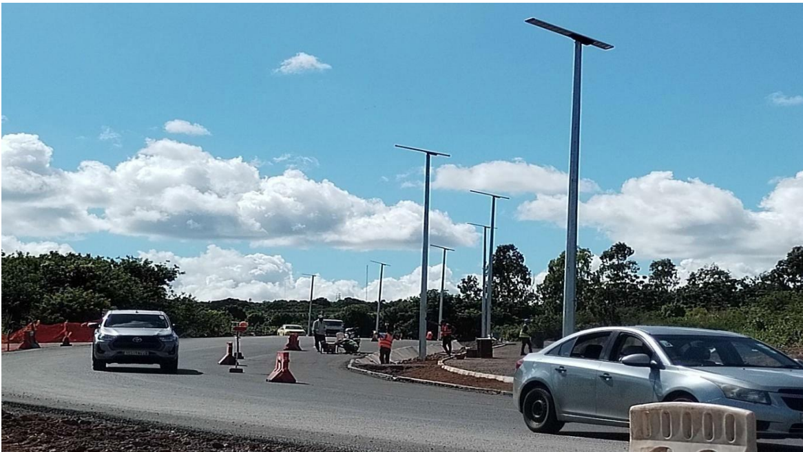
Upgrading of Part of Hollyrood Road
