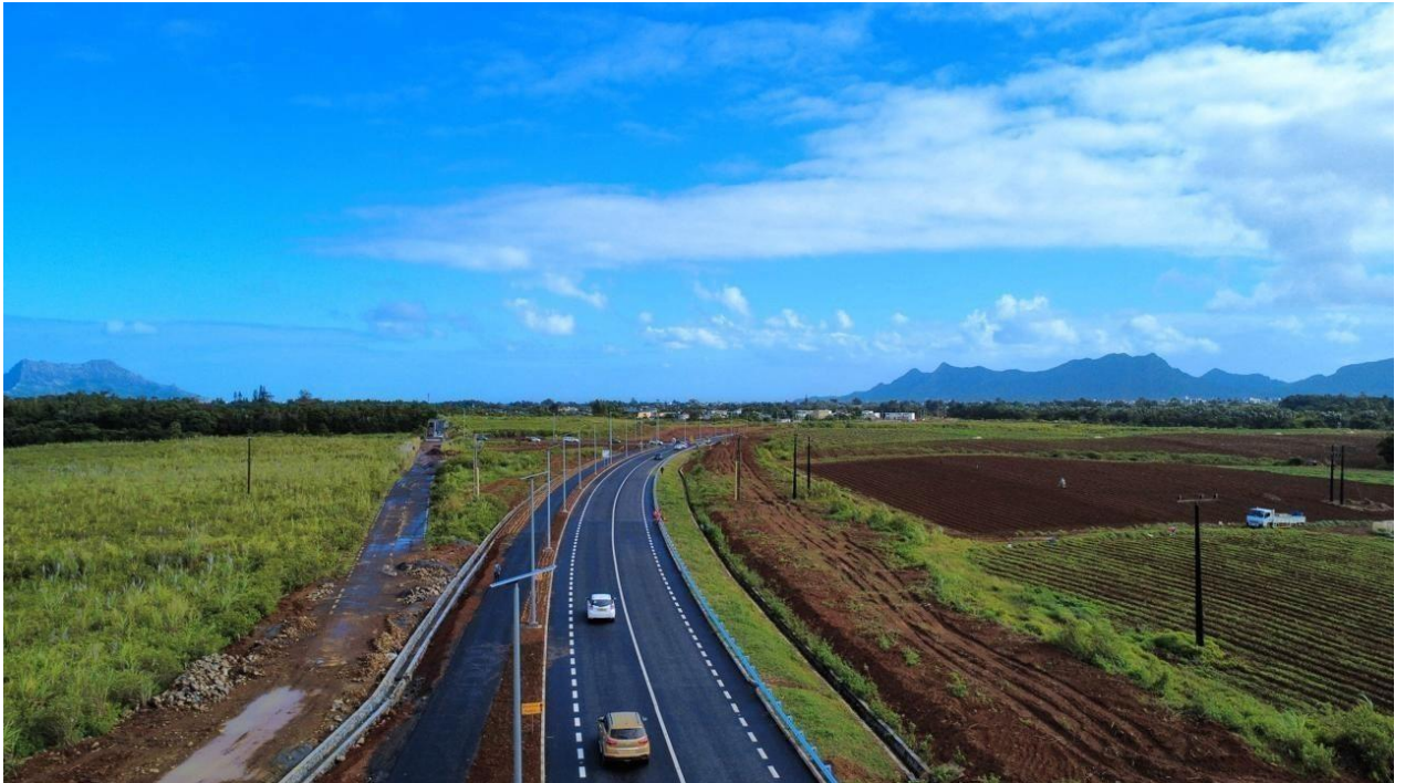
Construction of Hermitage Bypass
