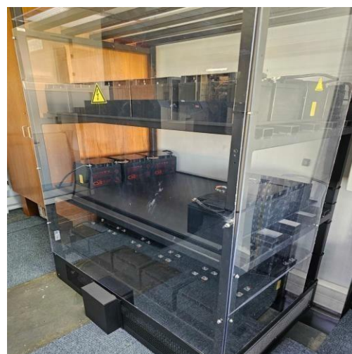
Fig 2: Battery Pack (30 mins)
