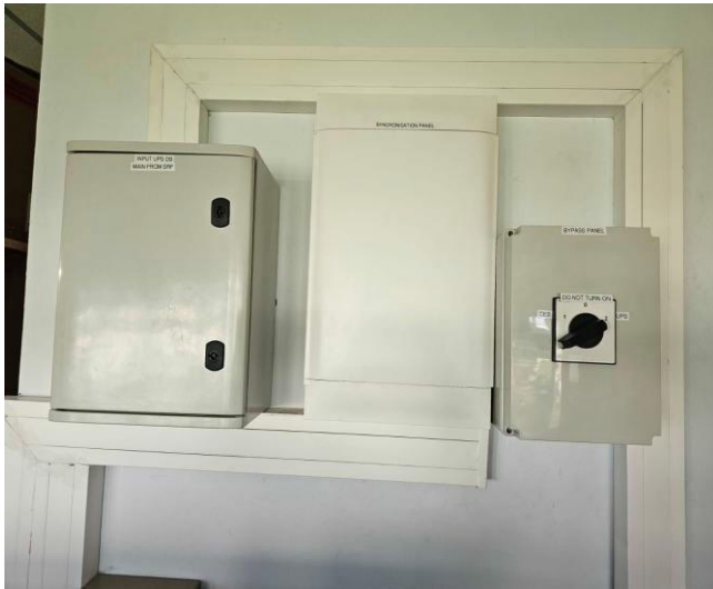
Fig 3: Input Panel for UPS
