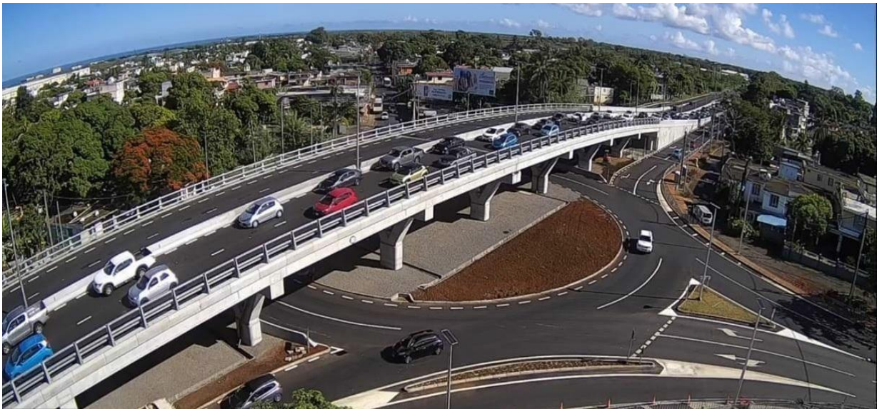
Construction of Flyover at Terre Rouge on Motorway M2
