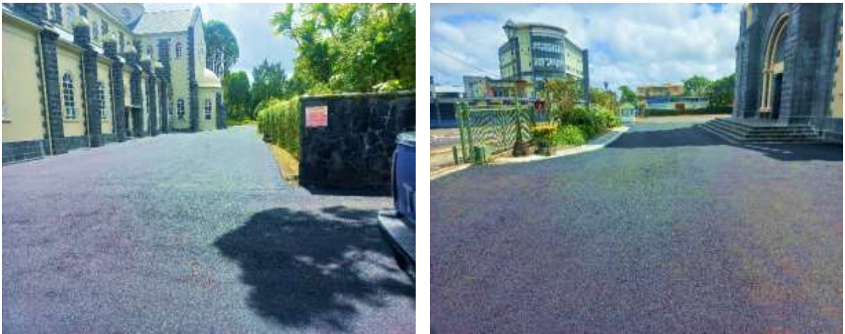
Figure 31: Embellishment Works and Resurfacing of Yard at Chapelle Notre Dame de Lourdes Curepipe
