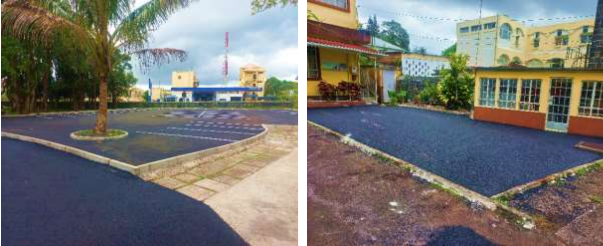
Figure 28: Enlargement of Access to Parking, Laying of Kerbs and Asphaltting works at Ste Therese Church
