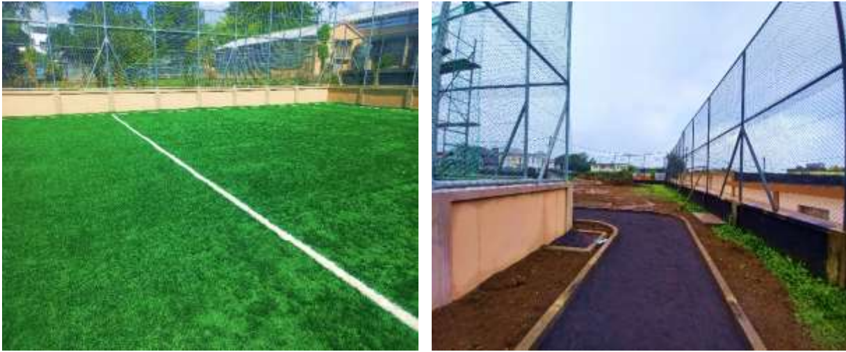
Figure 26: Construction of Mini Soccer Pitch and Jogging Track at Allée Brillant Floreal Football Ground
