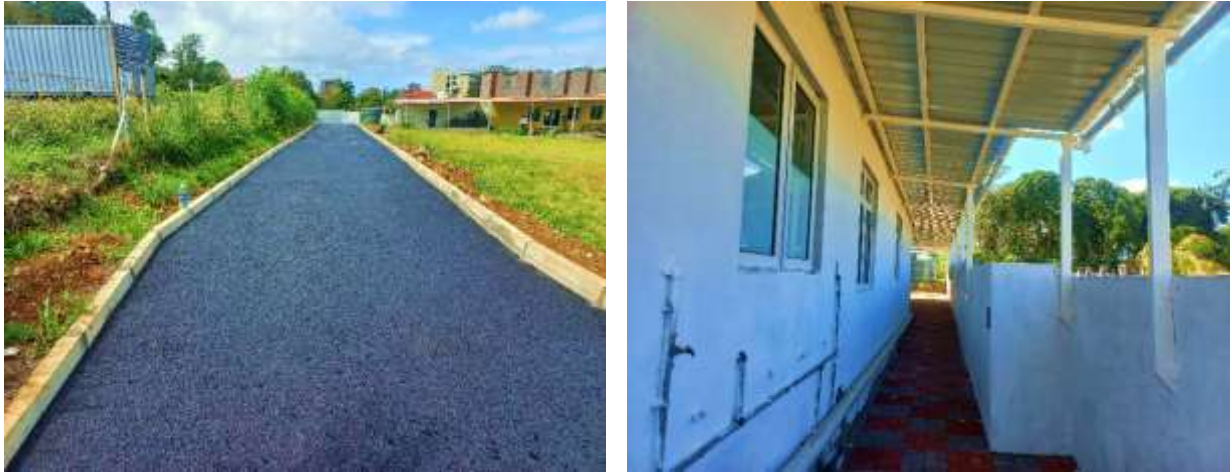
Figure 30: Tarring works, Laying of Interlacing Paviments and Construction of metallic shelter at Trianon Mariamen Temple Society
