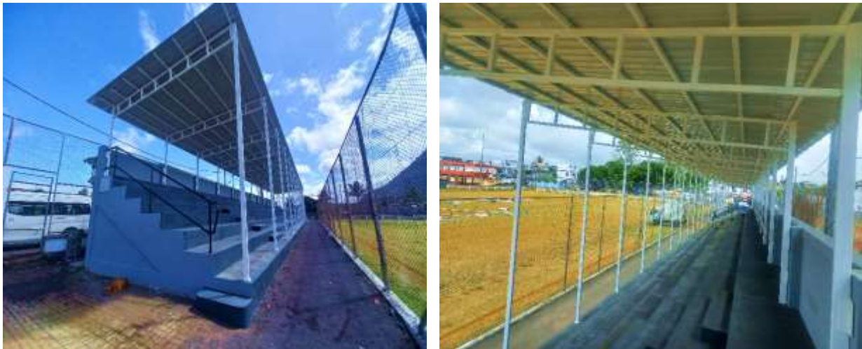
Figure 27: Painting, Reinstating Concrete Steps and Construction of Metallic Shelter at La Source Football playground
