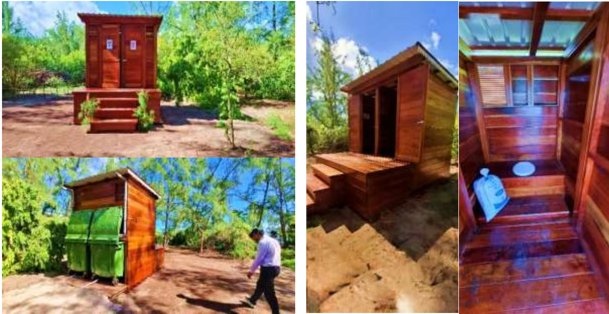
Figure 24: Construction of Dry Toilets at Ile aux Benitiers
